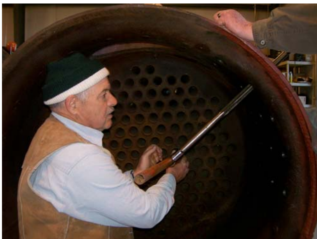
Bill tapping boiler for stay bolts
