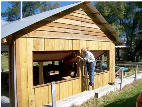
Steve installing redwood trim
