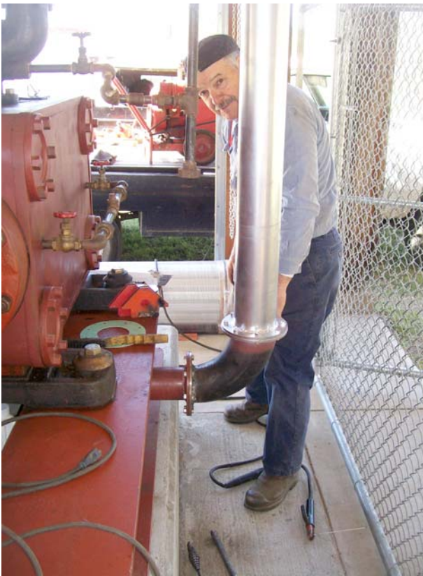
Bill and the new 5" exhaust pipe
