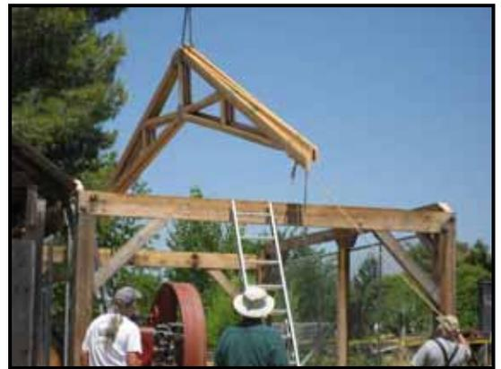
Before the fair opened, the Corliss was trucked to the sawmill and rolled onto its foundation using rollers, a come-along, and brute force. The flywheel was lifted by crane onto its foundation and carefully aligned with the Corliss. Only then could the trusses be placed over the new engine room and the new metal roof finished.
